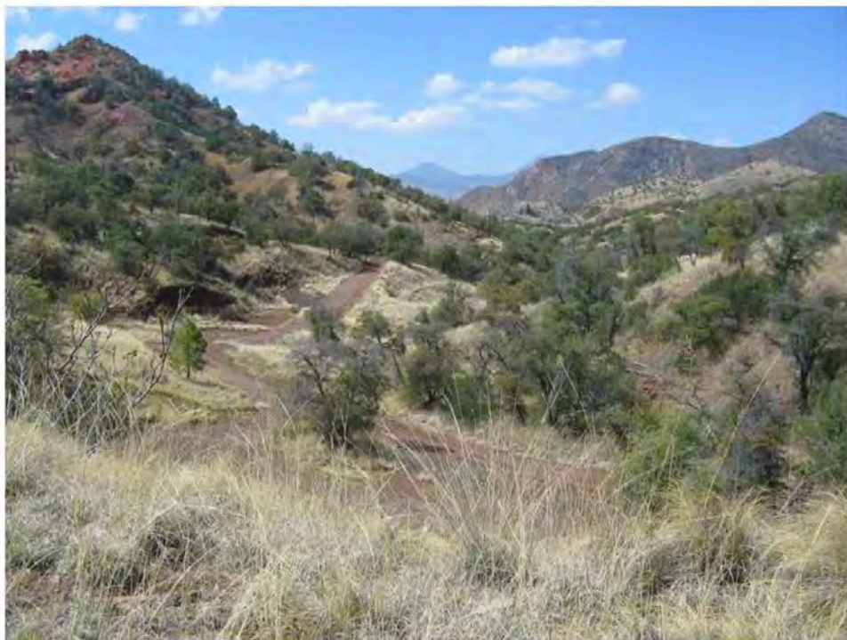
Looking down valley from catchment dam, below tailing pile no. 4. Note that terrain is too steep to accommodate an alternative site for the two evaporation ponds, each about one acre in size.
