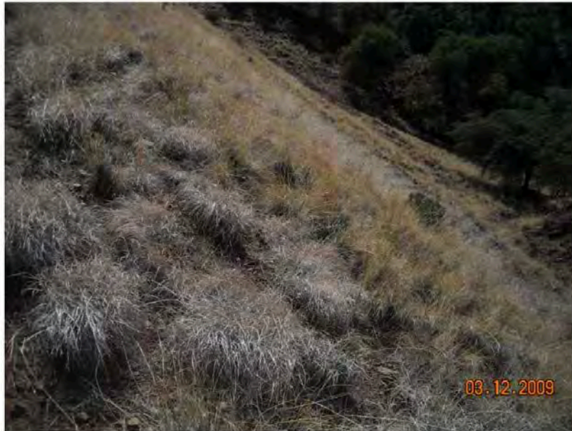
Close-up of side slope of tailings pile no. 4 showing the steep-sided nature of the tailings impoundments' slopes
