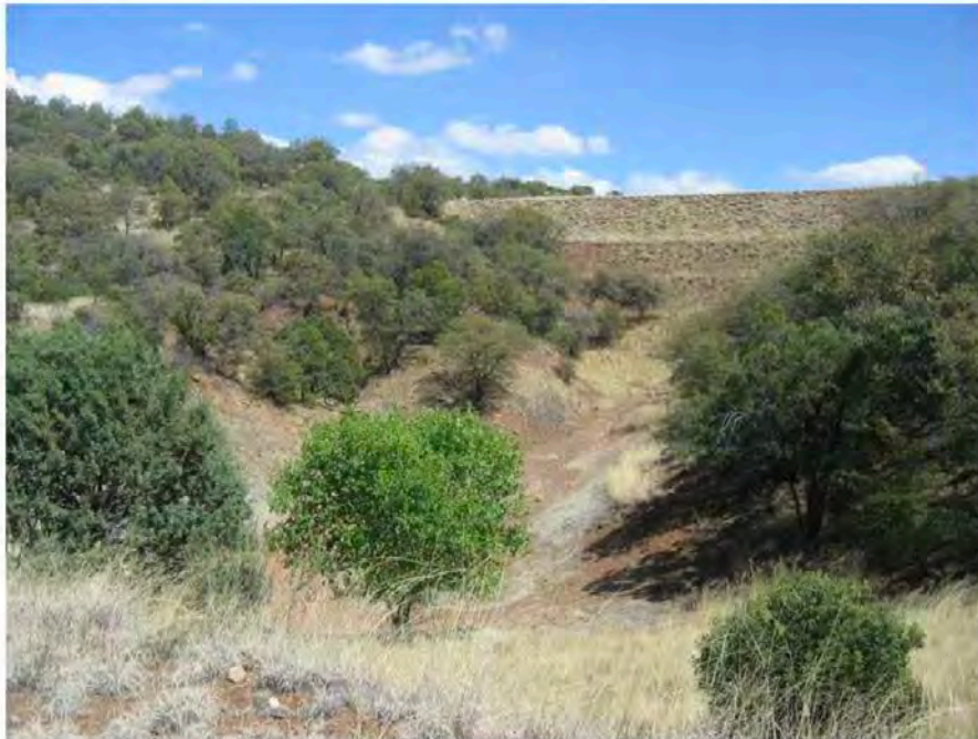
View of tailing pile no.4, looking upstream; this pile is the second and lowermost of the two piles proposed for installing the evaporation ponds. Note steep sided nature of this pile, showing the need for additional reinforcement (buttressing) to support additional weight of ponds
